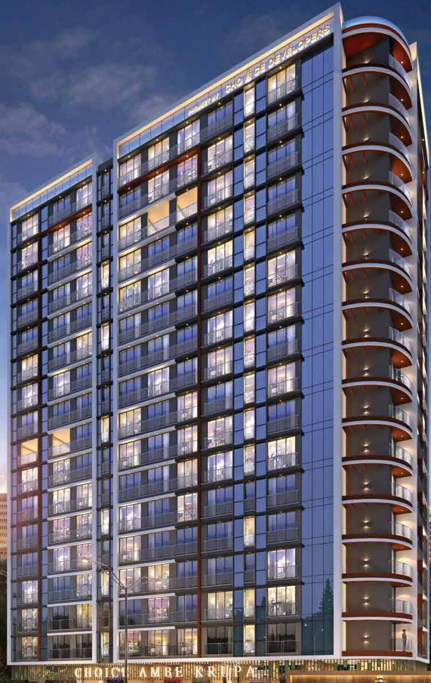
AMBE KRUPA BUILDING NO. 38
